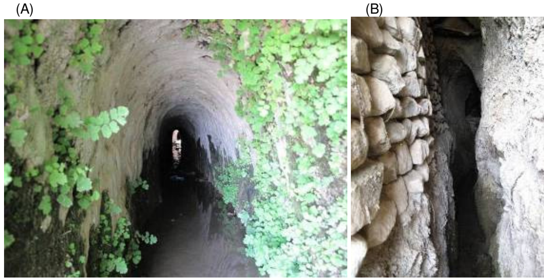
Figure 5. (A) Round arch karez tunnel in limestone at Zimzimuk; (B) Pitched and pointed arch Sarsula karez at Girdashekhal (in limestone). (Photos by Dale Lightfoot)
