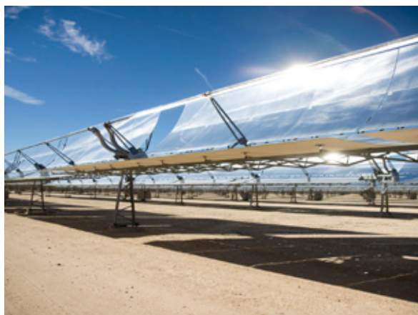
Solar thermal plant (parabolic trough).
